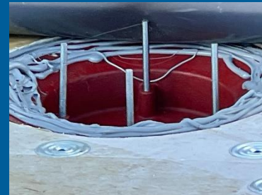
Roofing Activities ongoing Setting of Roof Drains
