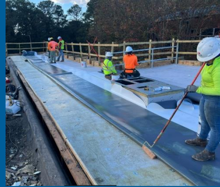
Roofing Activities ongoing Setting of Roof Drains
